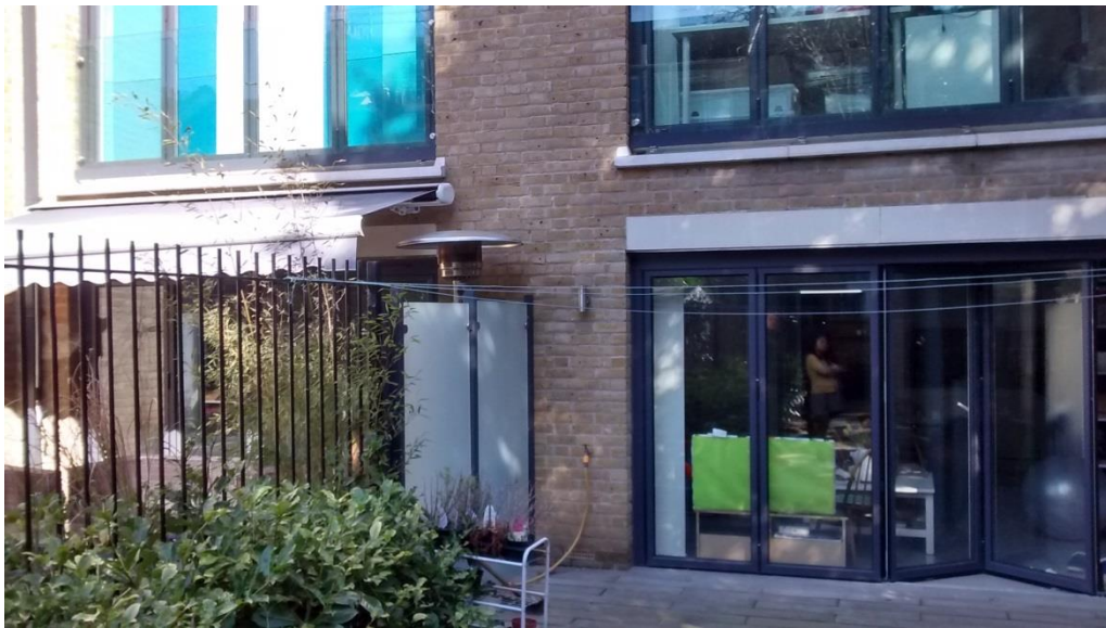
Image 2: Photograph of Rear of 7 Loxford Gardens toward 8 Loxford Gardens
